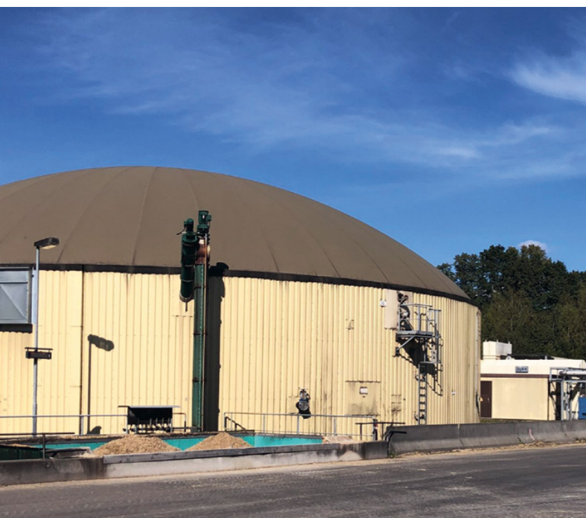
The biogas facility in Schöpstal acquired by BALANCE in 2022
